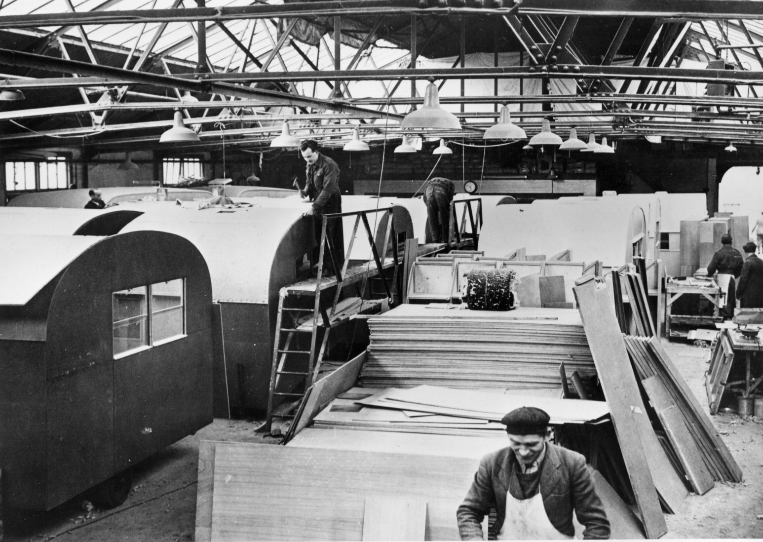
Newmarket Production line of 9ft Colts with PVC covered softboard roofs.
